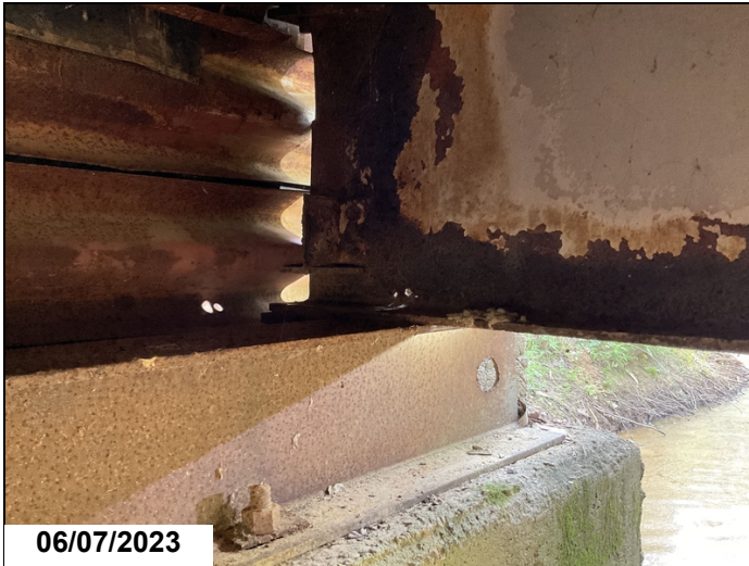
Section loss holes on beam 5 at bent 2
