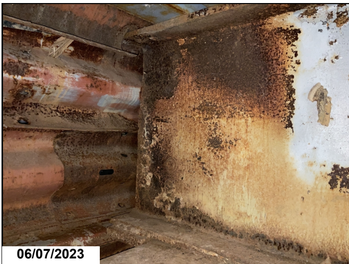
Beam 2 section loss @ bent 2
