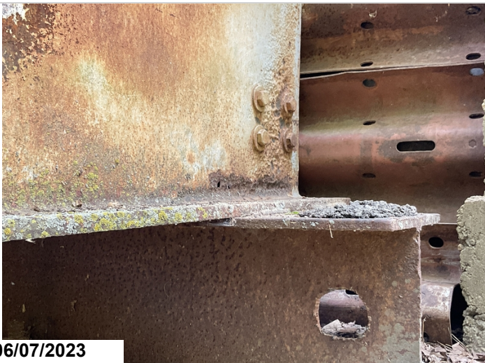
Bent 2, Beam 5, small holes in the beam; it's 13" from the end of the beam in the web area, CS3.
