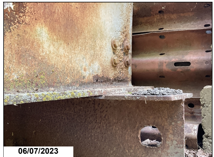
Beam 5 @ bent 2 has holes in beam. 13" from end of beam in web
