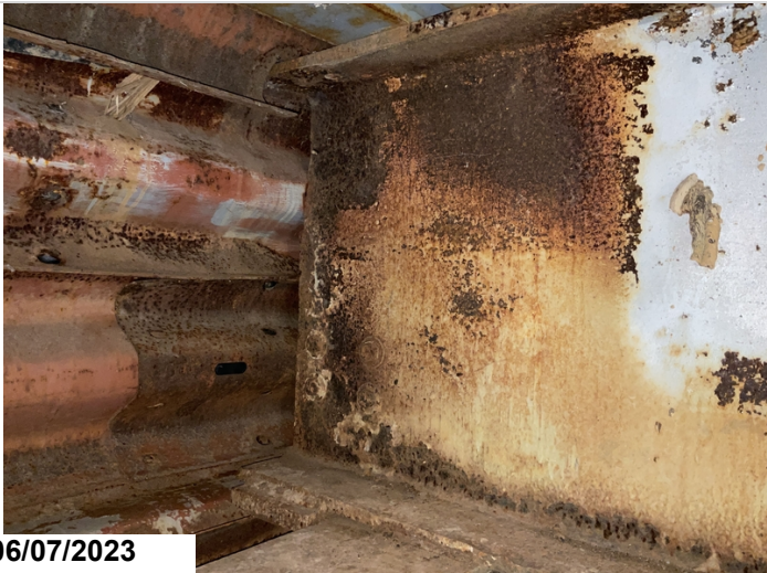
Bent 2, beam 2, section loss in various locations, CS3.
