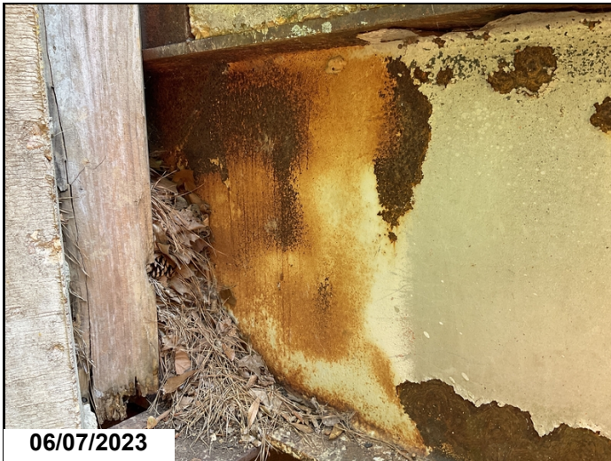
Corrosion to beam ends
