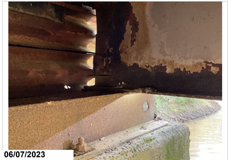
Bent 2, beam 5, small holes with minor section loss, CS3.
