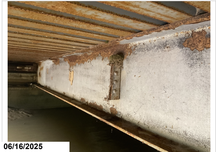
All steel beams have paint loss, CS2.
