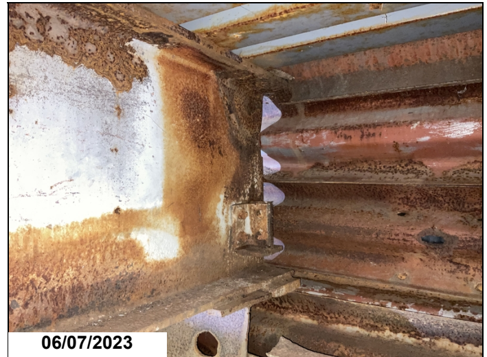
Beam 2 minor damage
