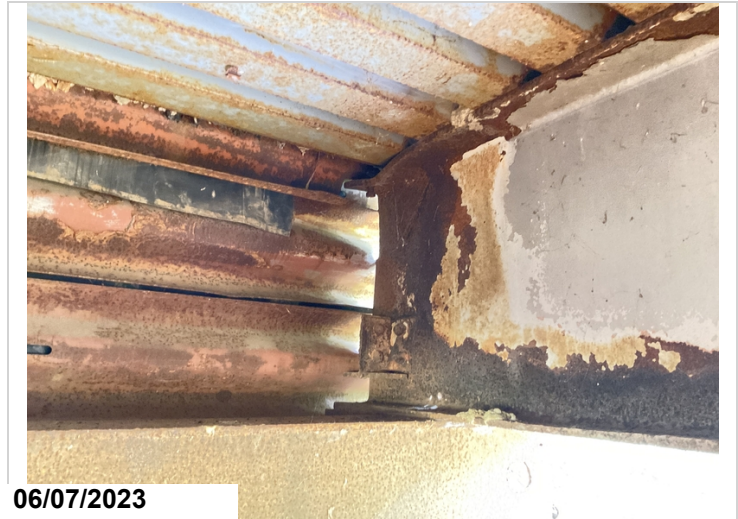
Bent 2, beam 5, The steel beam has damage, CS3.
